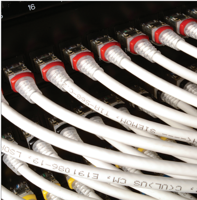
Within Wellstar's high-density copper patching areas, SkinnyPatch® Modular Cords improve manageability, airflow, and flexibility.
